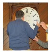
Great care must be taken when removing or reinstalling the dial - it's about  $\frac{1}{2}$  inch thick and very heavy. If damaged it is virtually irreplaceable.
